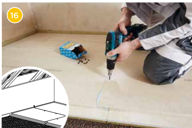
Connect the Rigidur flooring elements at the rebate edge with Rigidur drywall screws at intervals of approx. 25 cm.
