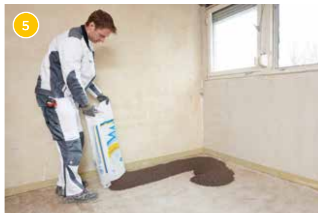
Place the levelling compound sack on the floor, cut it open at the bottom and lift the sack upwards. Then spread the compound on the floor space.
