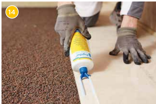
Apply the Rigidur Nature Line screed adhesive with the double-strand nozzle on the edge of the panel and on the rebate edges of the Rigidur flooring element.
