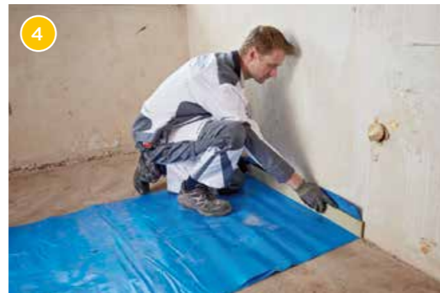
For concrete concrete floors directly bordering on the ground, lay a PE film with approx. 30 cm overlap. On wooden substrates we recommend permeable paper roll as trickle protection.
