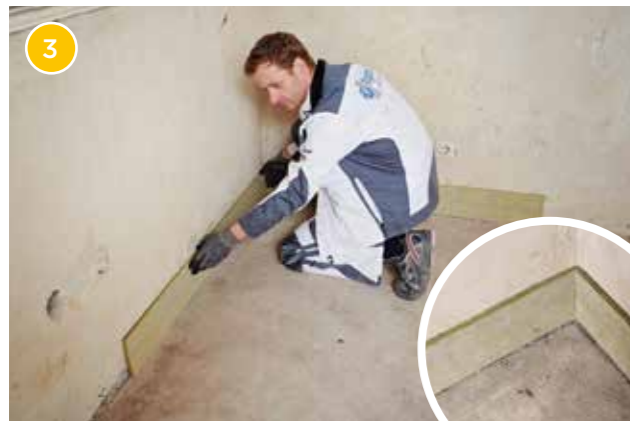
To avoid footfall sound transmission from floor to wall, lay a Rigips mineral wool edge insulation strip circumferentially. Pay particular attention to the wall corners.
