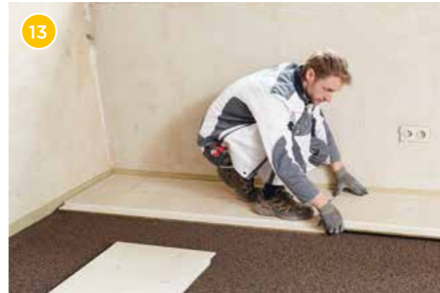
Lay the Rigidur flooring elements in rows longitudinally.
