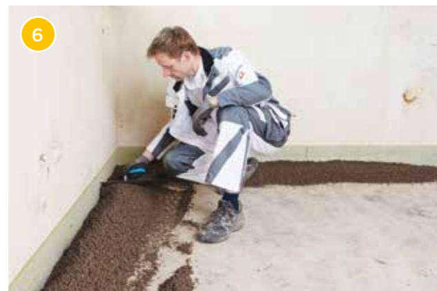
Level out unevenness and inclined floors with Rigips levelling compound. Levelling height: 10 to 100 mm.
