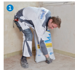
Cut the sack open at the bottom
