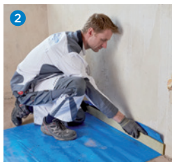
Laying out the film
