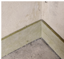
Attach edge insulation strips
