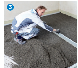
Smooth off using screed rails
