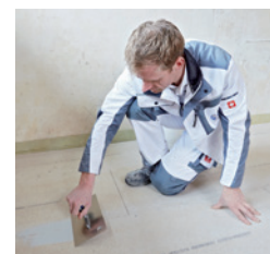
Filling of fastening points and any surface defects
