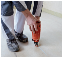
Fastening with expansion clamps
