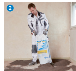
Carefully lift the sack upwards
